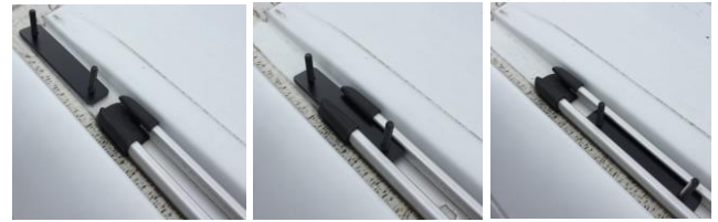
Figure 14: Track Threaded Insert Installation
