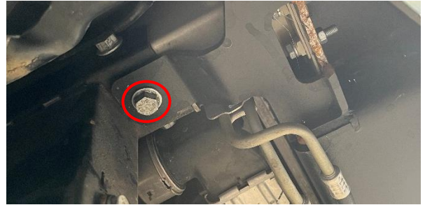
Figure 20: Installed Factory Crossmember Bolt Thru Winch Tray
