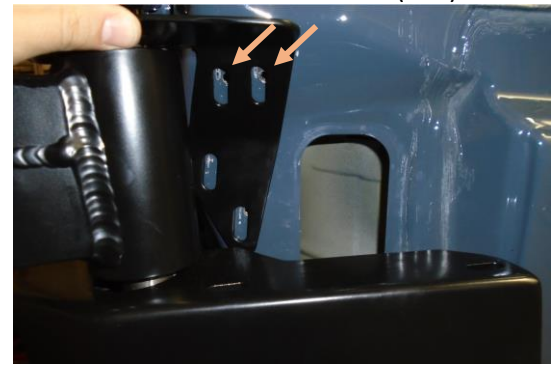
Figure 11: Drilling for Axle Support Bracket
