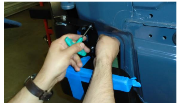
Figure 12: Tightening Hardware Through Insert Opening
