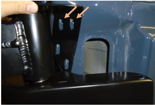
Figure 11: Drilling for Axle Support Bracket
