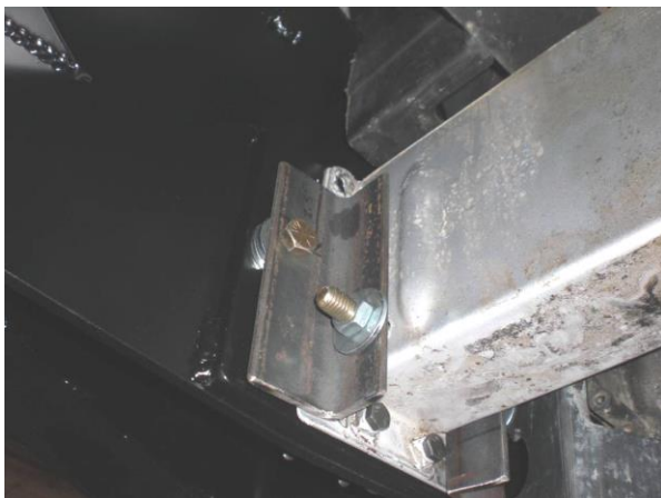
Figure 20: Steel support brackets bolted to frame
