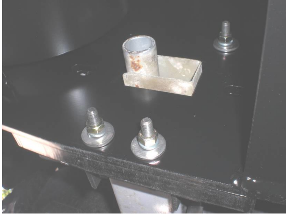
Figure 21: Frame mounting bolts with lock washers and 5/16" washers installed
